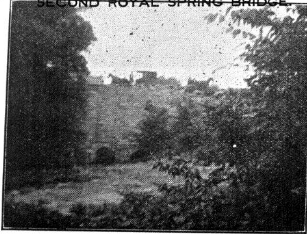
SHOWING VEHICLES ON FRANKFORT ROAD.
