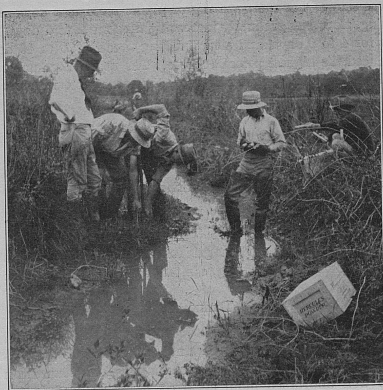
Placing dynamite on a curve in the ditch in the Elkhorn Creek drainage project in Franklin County.
