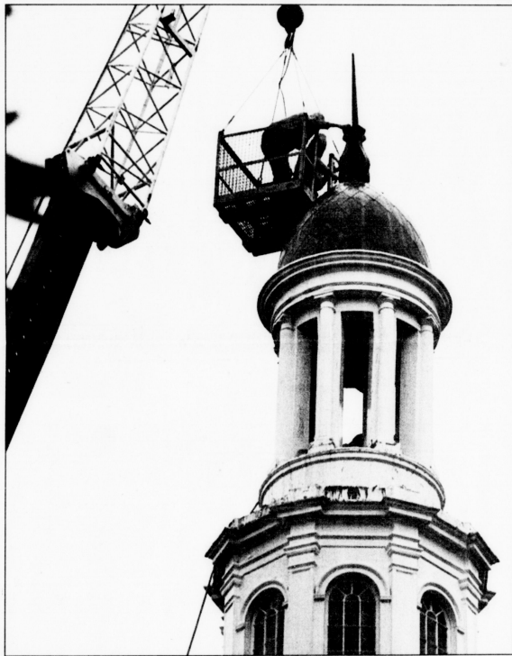
Workers repair Memorial Hall's steeple Friday afternoon. UK's signature building was struck by lightning and caught fire early Friday morning.
