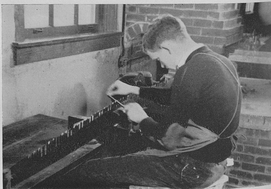
Sharpening a Crosscut Saw in the Shop
