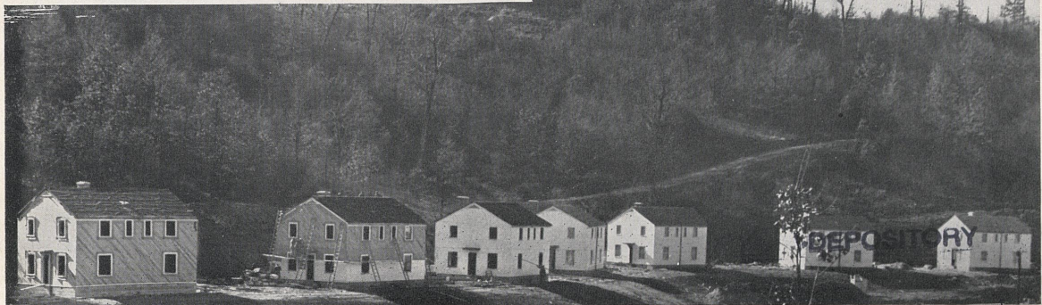
This housing project, which provides new homes for 70 low-income families, marks Mount Hope, W. Va., as one of the most progressive small towns in the country.
