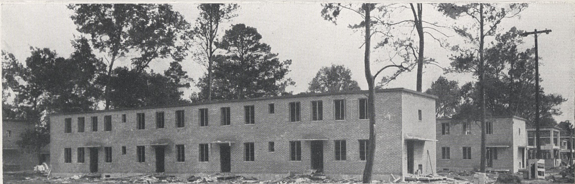
They will cost Uncle Sam less by nearly one-half. Dwellings under construction on the Cuney Homes project in Houston, Tex., where the Federal subsidy is only 1.862% of development cost; legal maximum subsidy is 3.5%.
