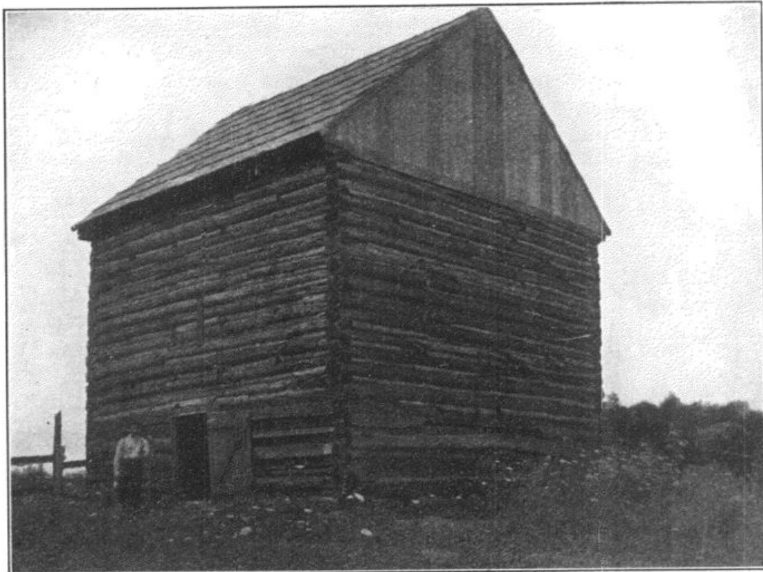
FIG. 13.—Common type of Virginia log barn for curing dark tobacco with open fires. (Photographed by the Bureau of Soils.)
