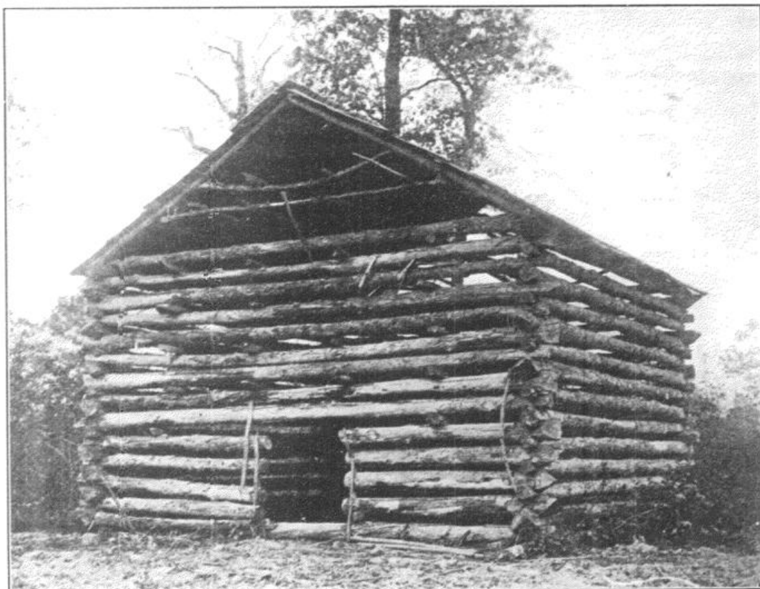
FIG. 9.—Early type of log curing barn for air-curing tobacco still seen in some of the Virginia, Kentucky, and Tennessee districts.
