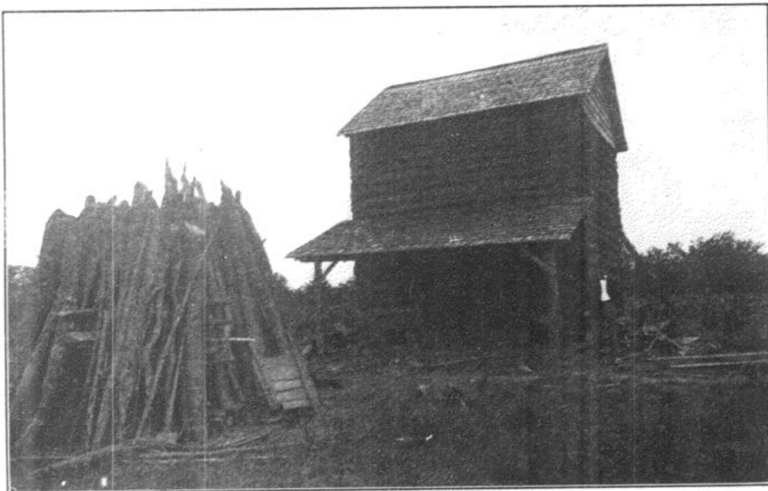
FIG. 24.—Typical flue-curing tobacco barn, Old Belt section, Pittsylvania County, Va. The pile of wood is for burning in the furnaces.
