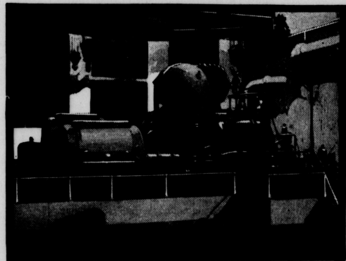
45,000 K. W. Westinghouse Cross-Compound Turbine Unit at the Station of the Narragansett Electric Light Company, Providence, R. I.
