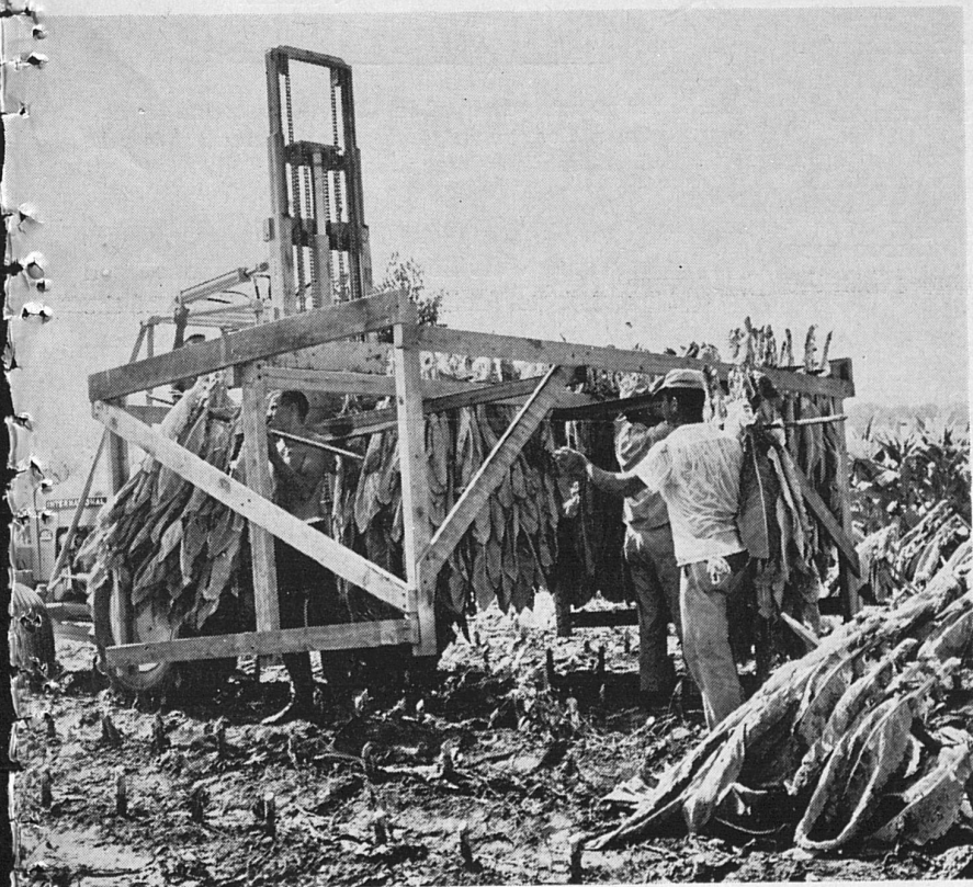
Field workers on a central Kentucky farm placing sticked tobacco into open loading frames. The fork-lift attachment on the tractor (left background) enables the operator to haul the loaded frames to the curing barn and stack them atop each other. If successful, the system would eliminate much of the customary barn labor and would also reduce safety hazards associated with housing tobacco.
