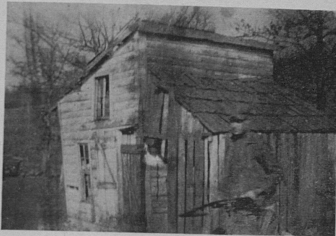
After the Poultry Specialists' Visit—Ready to Remodel the Old House.
