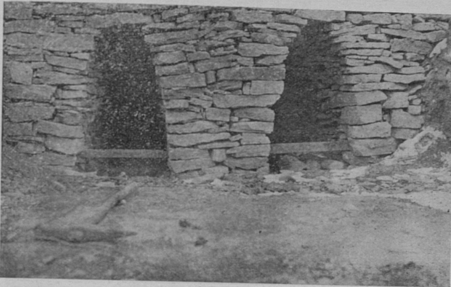
Front View of Limekiln showing "Eyes."
