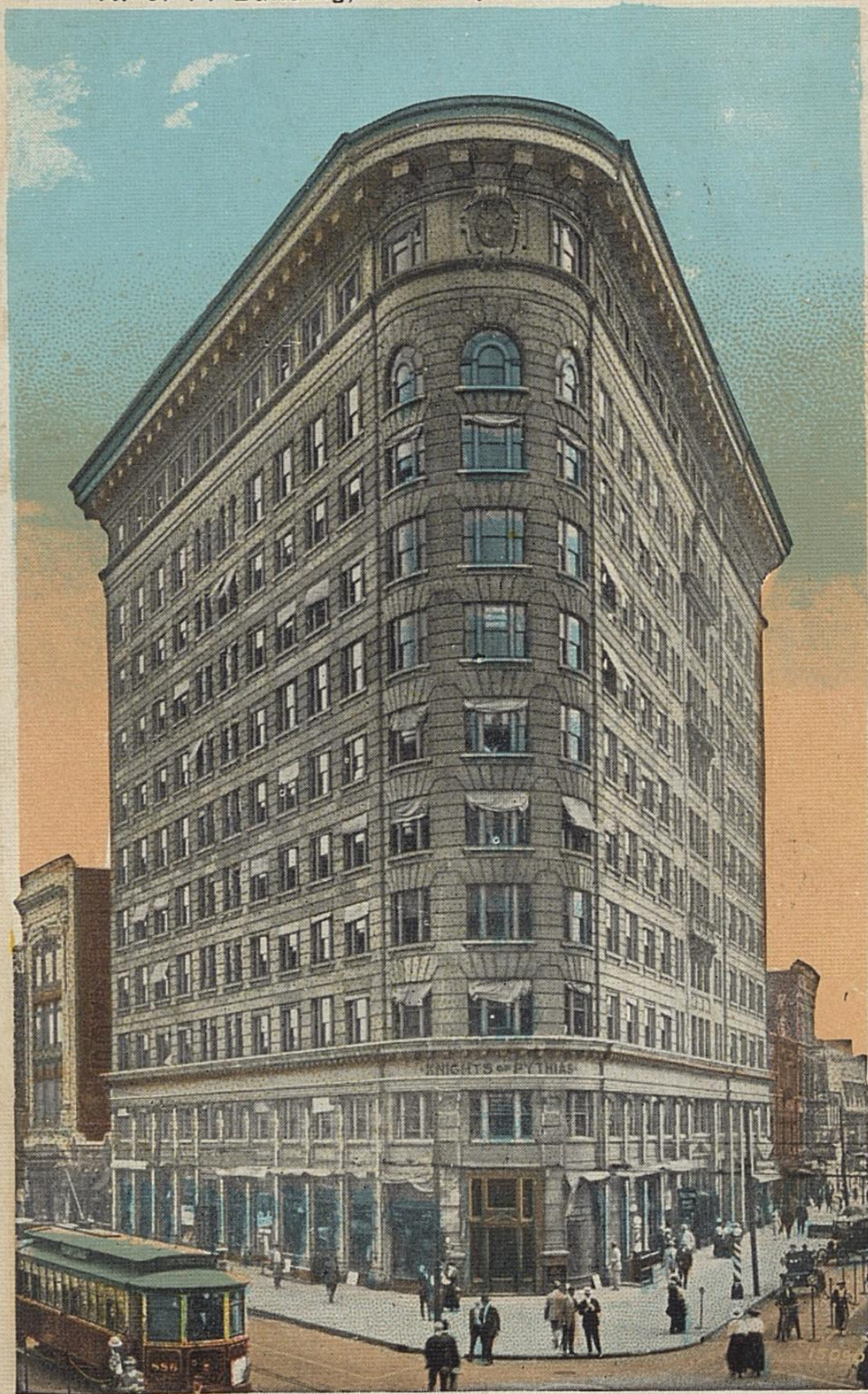
K. of P. Building, Indianapolis, Ind.
