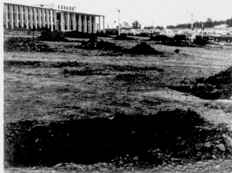
From the appearance of large holes in the ground around the Complex, one might think giant sized moles were having a field day. But, the holes were really dug in preparation for planting trees and shrubs in the area.
