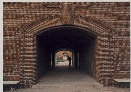
Brick detail-Engineering Quadrangle
