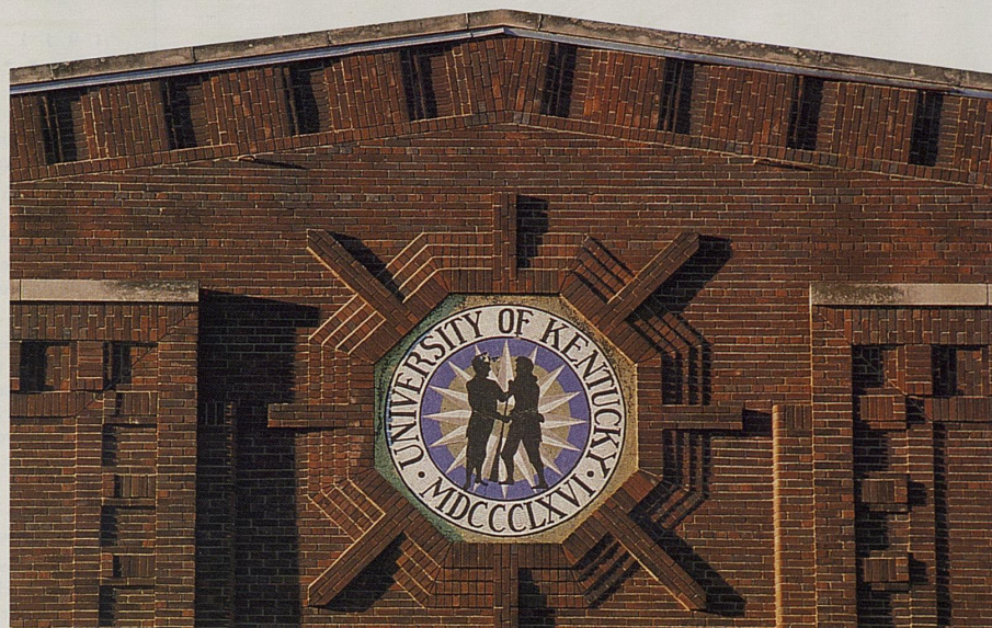
Brick detail-Funkhouser Building
