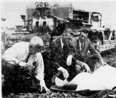
Ground breaking for the Agricultural Science Center gets underway as President Frank G. Dickey reviews the plans with Mr. David Pritchett, chief engineer for the state Department of Finance; Dr. Bennett H. Wall, associate dean of the College of Agriculture and Home Economics; and Robert Matthews, state Commissioner of Finance.
