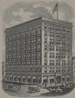
TRUST COMPANY BUILDING.
