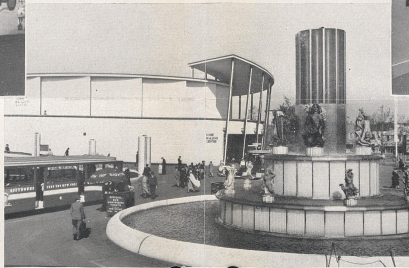
Above. The Dance of the Dams Fountain at Bowling Green in the World's Fair of 1940, in New York, with Home Building Center in background.
