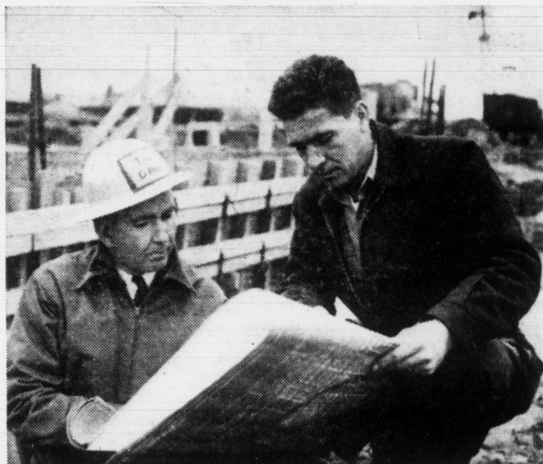
Cliff Downer (right), A.B. in Mathematics, '49, M.S. in Civil Engineering, '50, Harvard, on the site of a building construction project.
