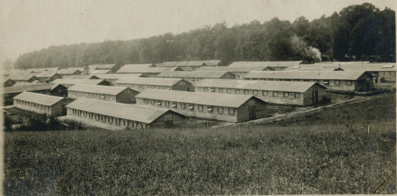
Hospital at St Mennhould. France.
