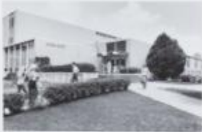
View of the Administration Building from the East
