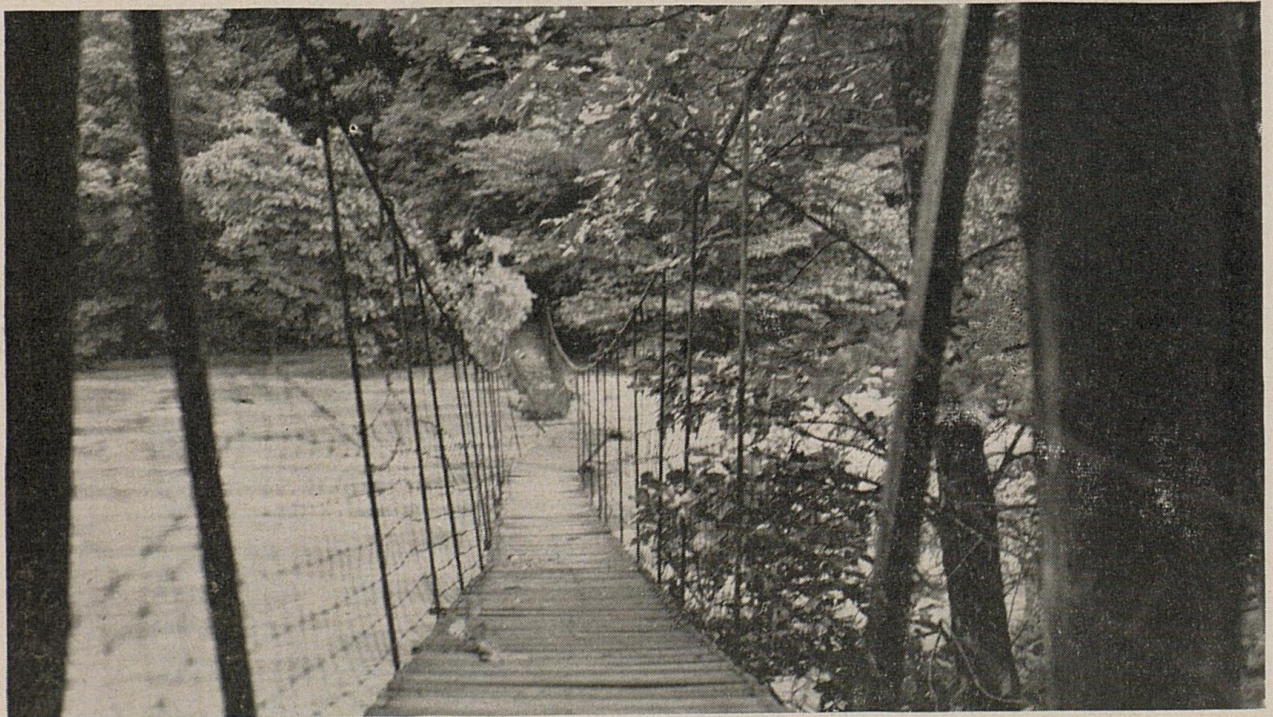
WENDOVER SWINGING BRIDGE WHEN FLOORING BEGAN TO BREAK
