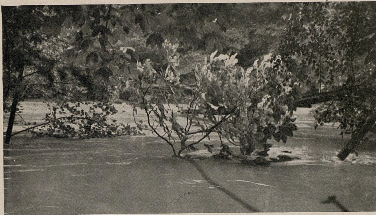
WENDOVER SWINGING BRIDGE AFTER FLOORING HAD GONE
