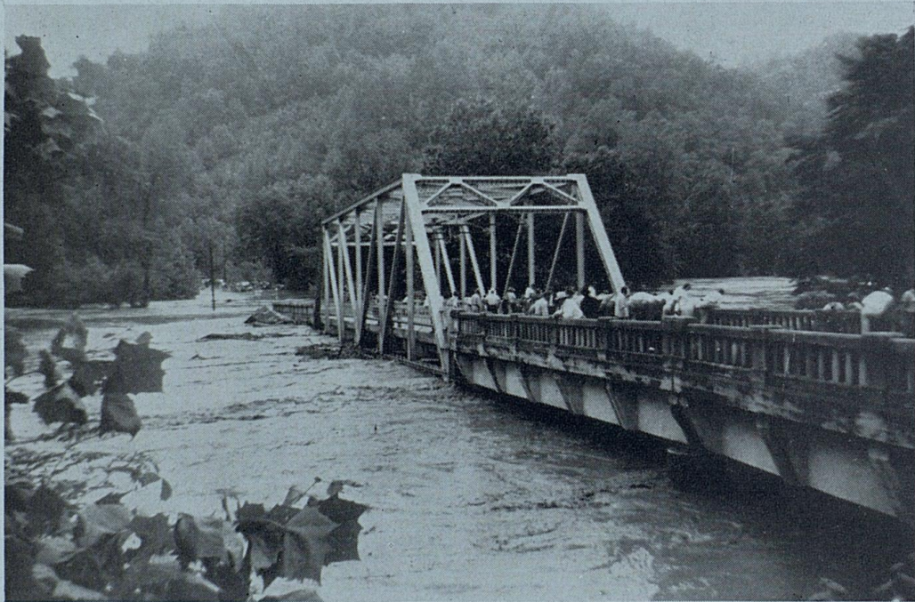
APPROACH TO HYDEN, BRIDGE OVER THE MIDDLE FORK IN THE JUNE FLASH FLOODS
