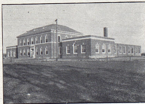
AGRICULTURAL ENGINEERING BUILDING
