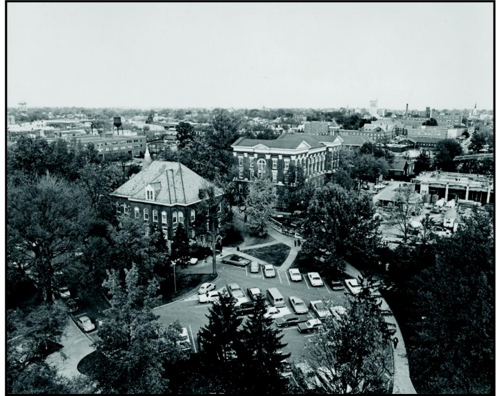
Patterson Office Tower, the most striking of several new structures that redefined the central campus area in the mid-1960s, is under construction in the upper right side of this image. POT was completed in 1968 and named for James K. Patterson, president of the university from 1869-1910. Along with the adjoining White Hall Classroom Building, it was built on the site of White Hall, one of the original State College buildings. It primarily houses faculty offices and conference rooms, including many of the offices of the College of Arts and Sciences.
