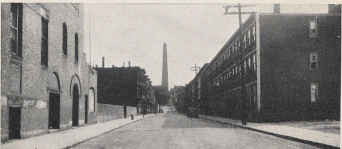
Boston, Mass. Nearly a thousand slum dwellings were demolished on this site to make way for the Charlestown project.
