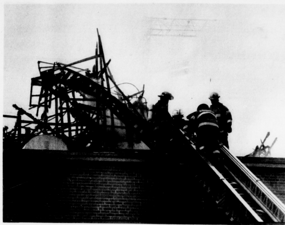
Firemen look at the damage to the UK Medical Center cooling tower after a fire damaged the top layer of the structure last Monday afternoon.
