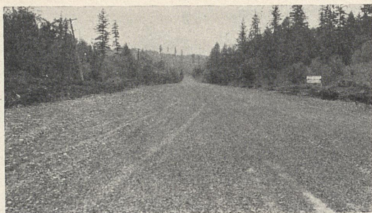
FIGURE 9.—COMPLETED ROAD. PICTURE SHOWS ABOUT THE SAME SECTION AS IN FIGURE 1.
