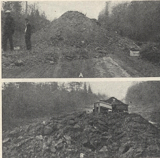
FIGURE 4.—FILL MATERIAL PILED ON ROAD PRIOR TO UNDER-FILL BLASTING. A, MATERIAL FROM UPPER 12 FEET OF BORROW PIT; B, MATERIAL FROM LOWER PART OF BORROW PIT.
