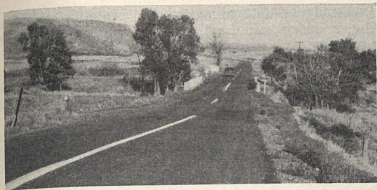
VIEW TAKEN FROM CREST OF HILL. NON-DIRECTIONAL MARKING RESTRICTS PASSING DESPITE ADEQUATE SIGHT DISTANCE.
