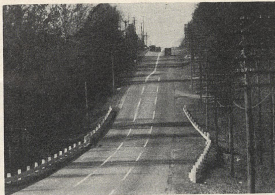
THREE-LANE HIGHWAY MARKED TO RESTRICT TRAFFIC TO TWO LANES OVER THE CREST OF A HILL WHERE SIGHT DISTANCE FOR UP-HILL TRAFFIC IS RESTRICTED. SUCH NON-DIRECTIONAL MARKING UNNECESSARILY RESTRICTS DOWN-HILL TRAFFIC WHICH HAS ADEQUATE SIGHT DISTANCE FOR PASSING, THUS ENCOURAGING DISREGARD FOR RESTRICTIVE LINE AND PASSING AS SHOWN.
