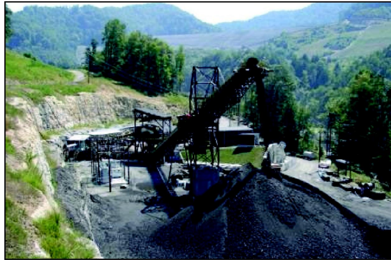
McCoy Elkhorn Coal Corporation, Mine #15, Pike County, KY.
