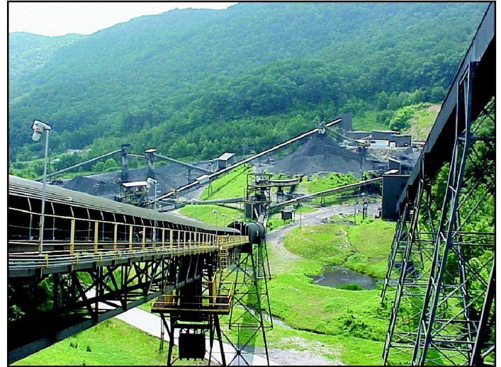
Clover Loadout, Bledsoe Coal Corporation, Harlan County, KY.
