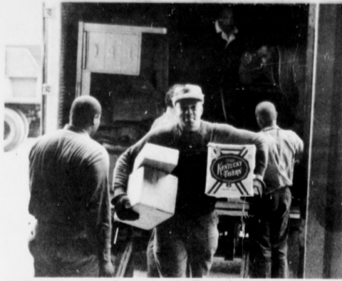
Workers are moving furniture and office supplies from White Hall offices to the old Agriculture Science Building. White Hall is one of three buildings scheduled for razing in early March to make way for the new office-classroom complex.
