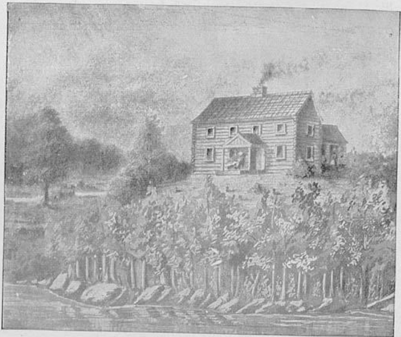
RESIDENCE OF GENERAL CLARK AT CLARKSVILLE.
