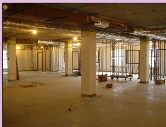
Third floor of King Building renovation.
