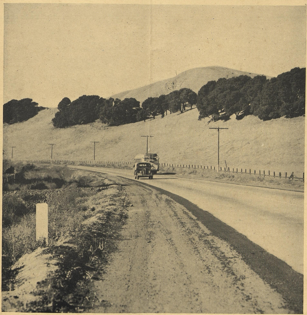
A SECTION OF STATE ROUTE 37 IN CALIFORNIA
