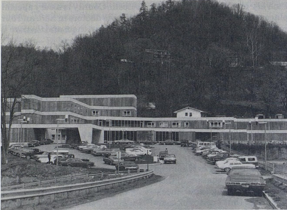
The Mary Breckinridge Hospital.
