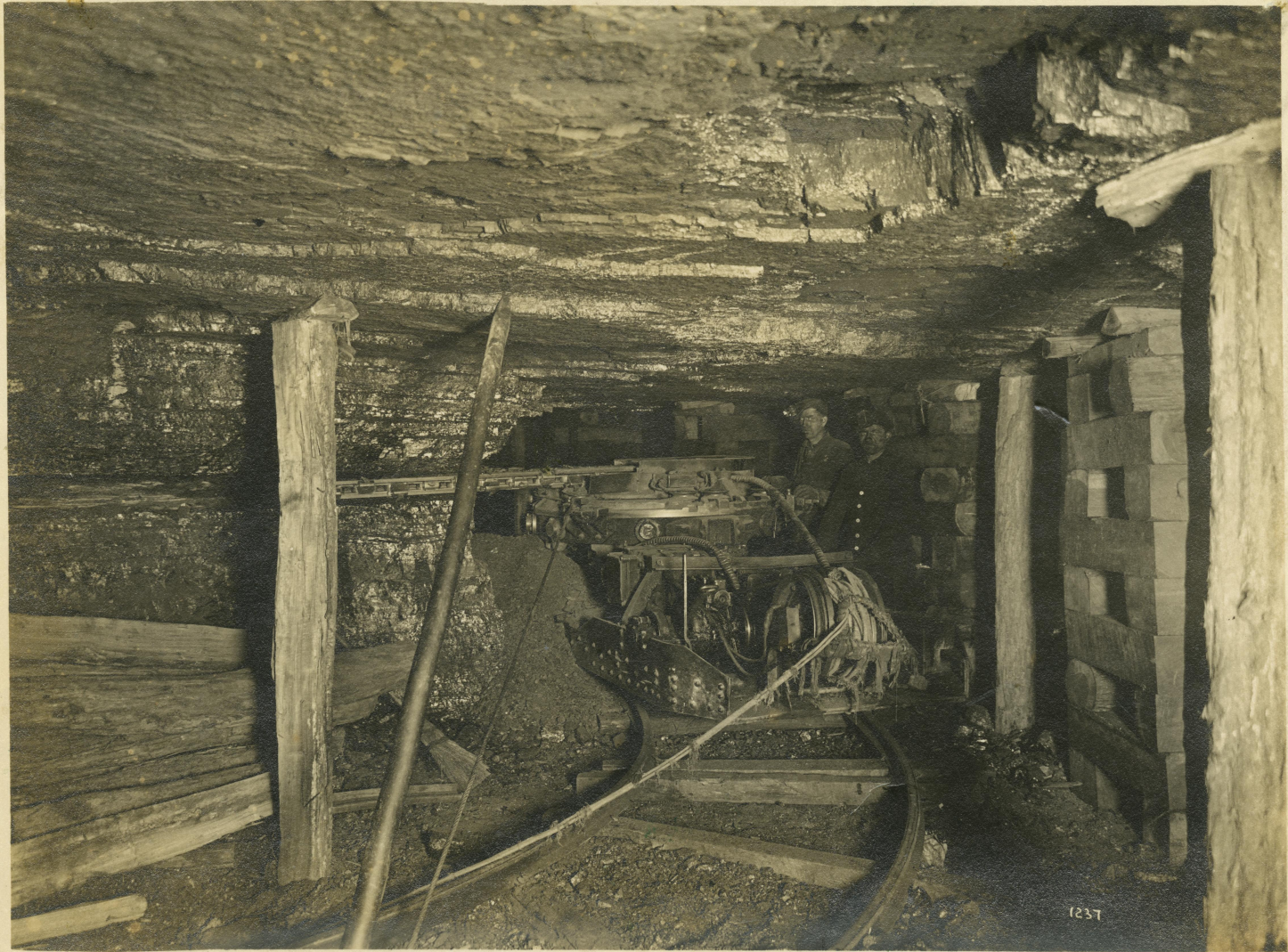
Longwall machine finishing cut ~ No. 204 Mine ~ Jan. 10, 1916
