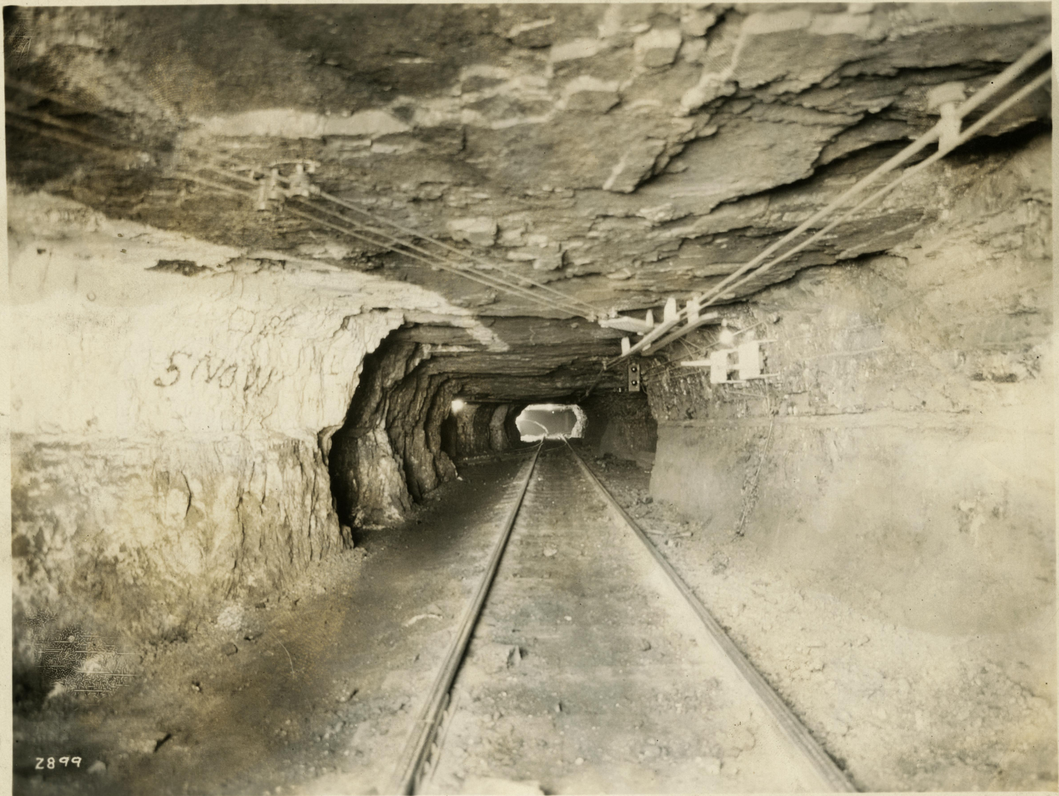
Main Line, 206 Mine ~ Jan. 10, 1930
