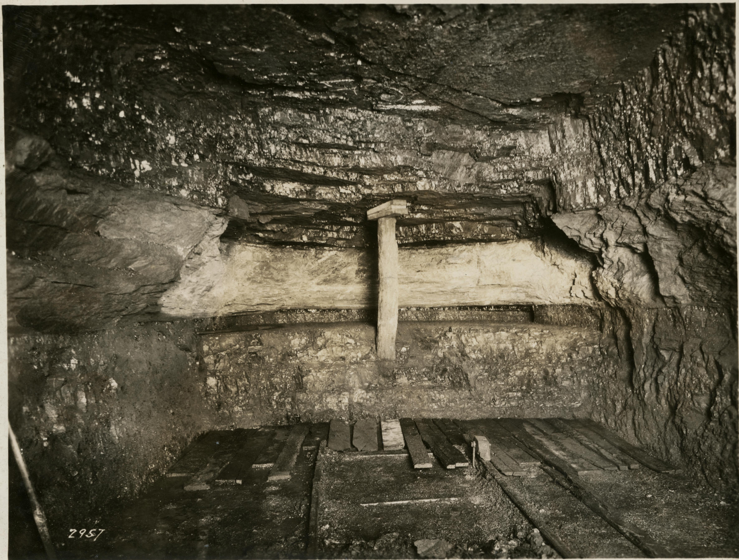
Parting Cleaned and Ready to Shoot ~ May 6, 1930
