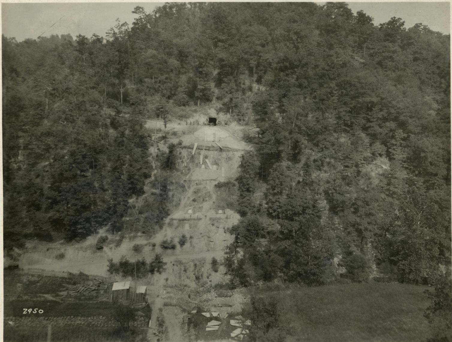
Progress on Kentucky River Bridge ~ Sept. 7, 1930
