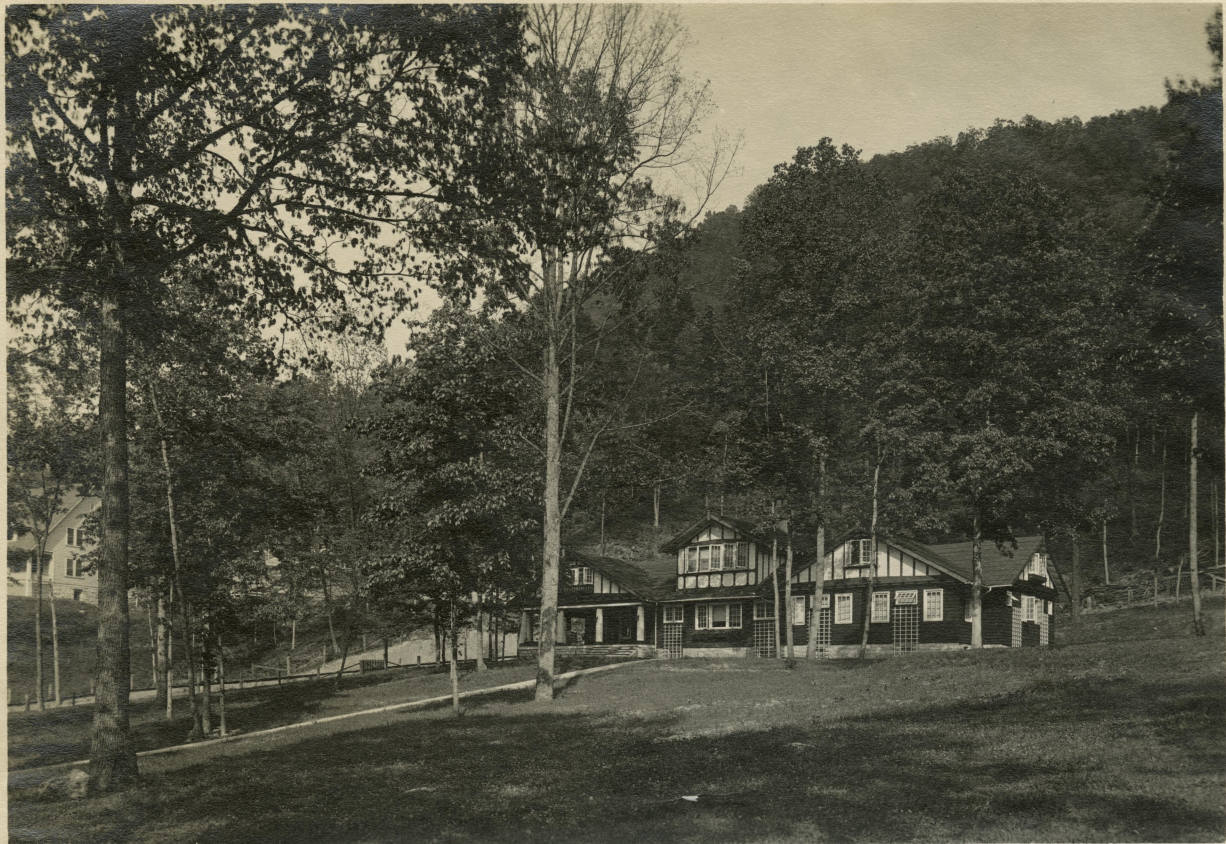
Manager's Residence ~ May 23, 1914
