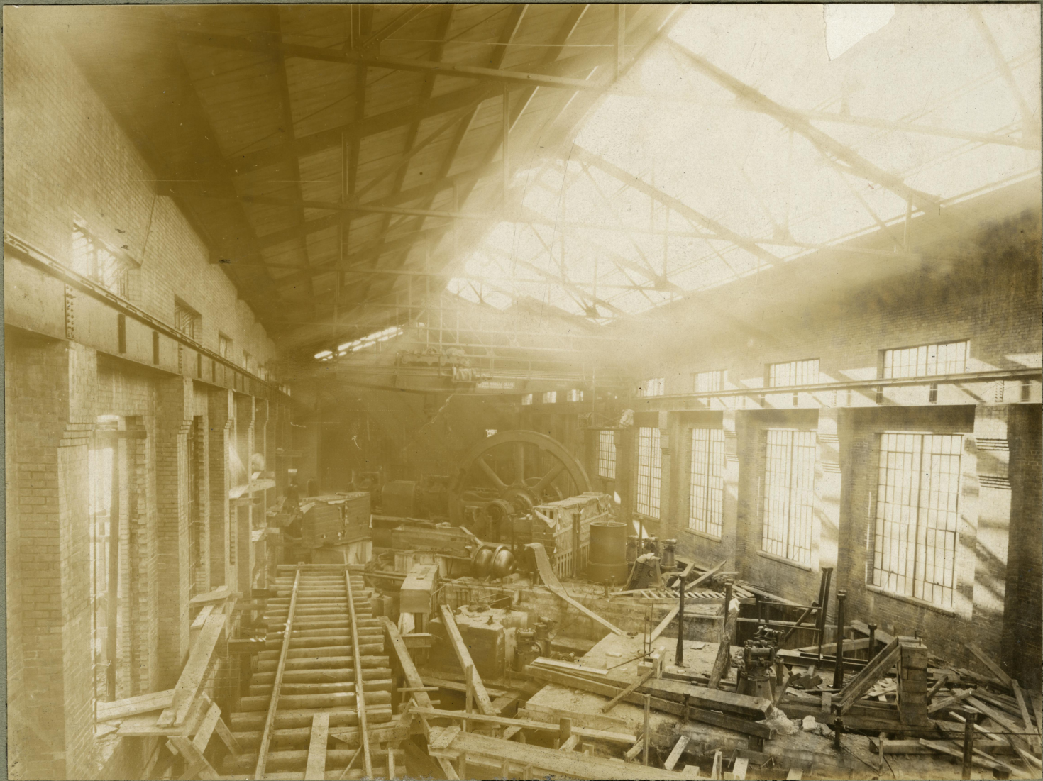
Interior View ~ Jan. 10, 1915
