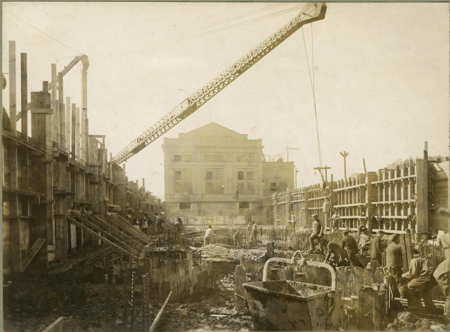
Concrete Foundation ~ Oct. 26, 1914
