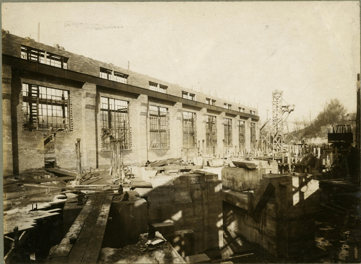
Engine Foundation ~ Dec. 12, 1914
