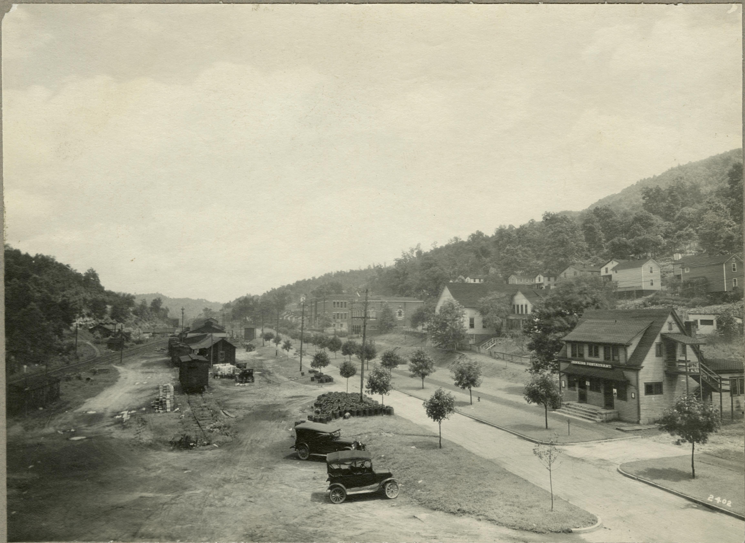
Main Street, Jenkins, KY, looking East from warehouse ~ Aug. 23, 1923
