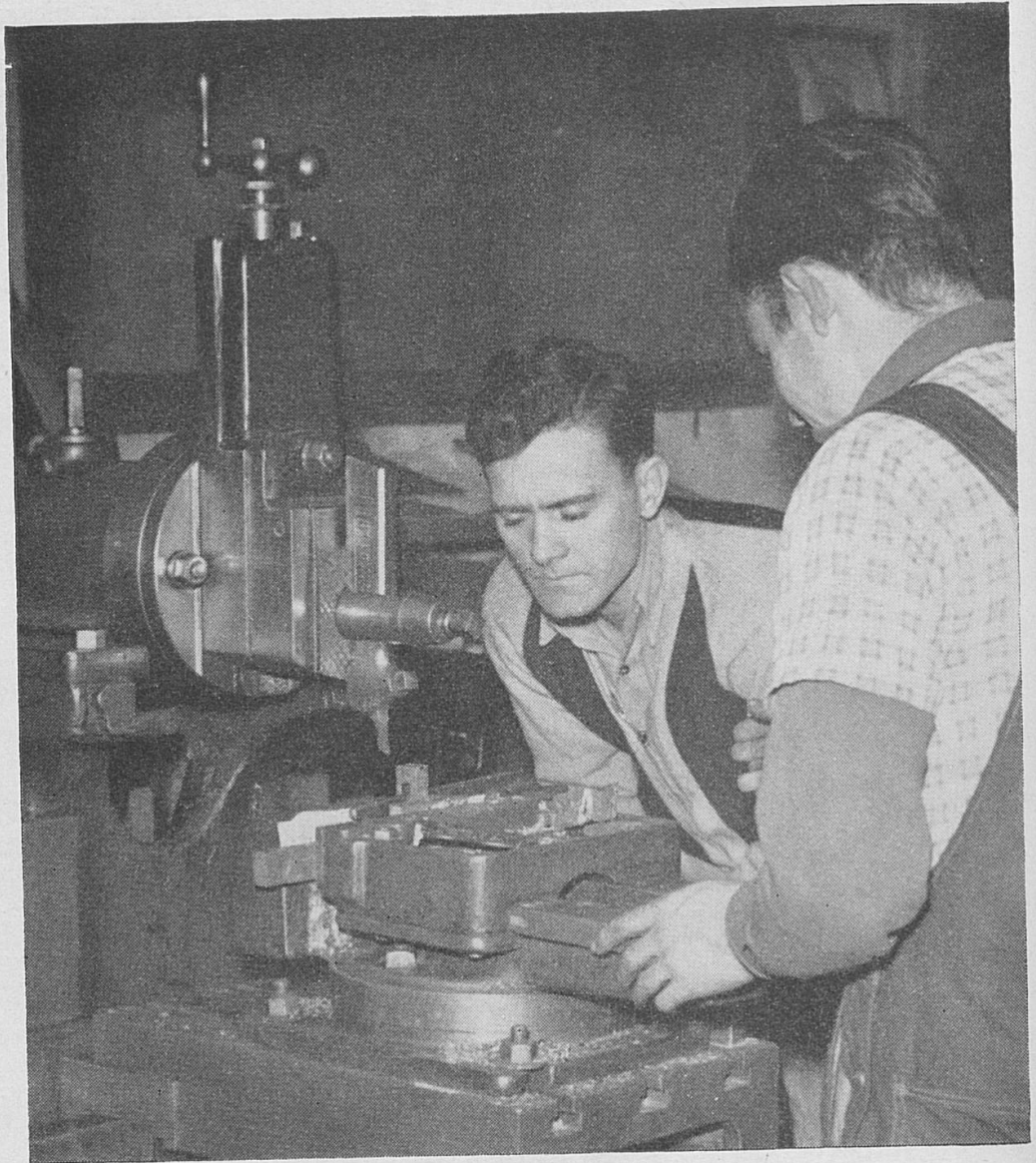
MACHINE SHOP CLASS Dressing a piece of steel on the shaper.
