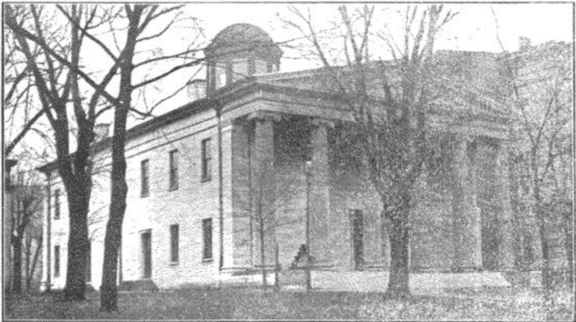
KENTUCKY CAPITOL. Of Kentucky marble. The cross in the lower right hand corner shows where Goebel fell. Several tragedies have occurred in this historic building.
