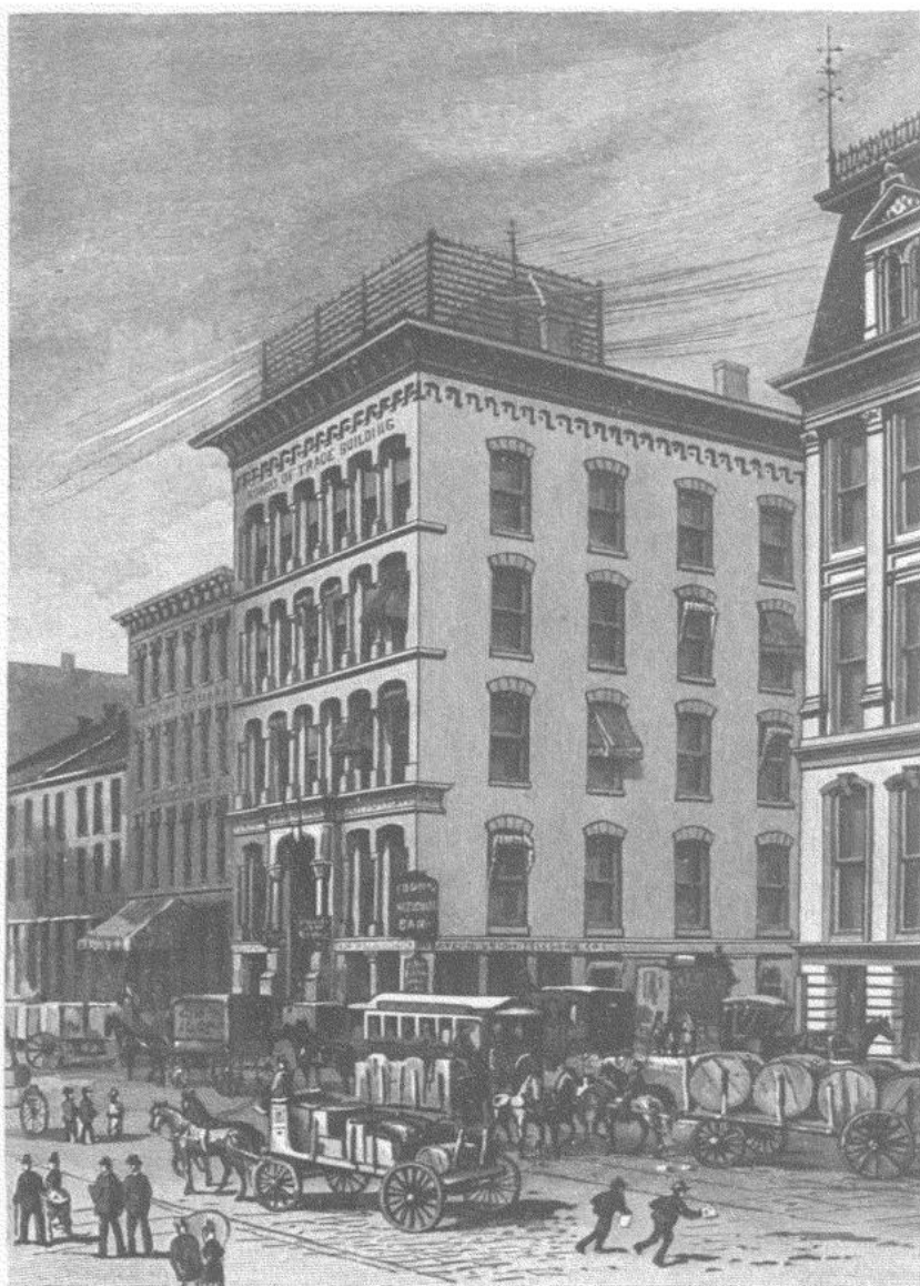
LOUISVILLE BOARD OF TRADE BUILDING.
