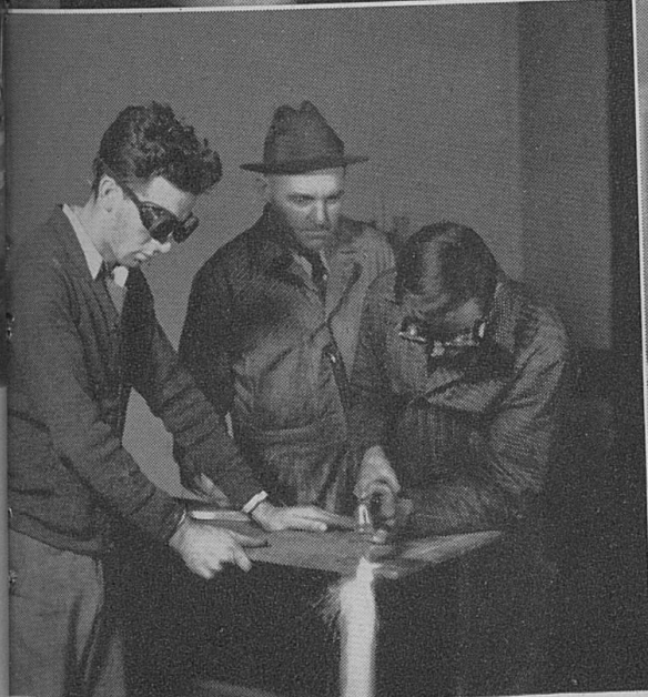
Cutting the Way Through a Tough Job.
