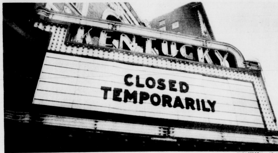
Most of the damage done to the Kentucky Theatre was mostly smoke-and-water damage.
