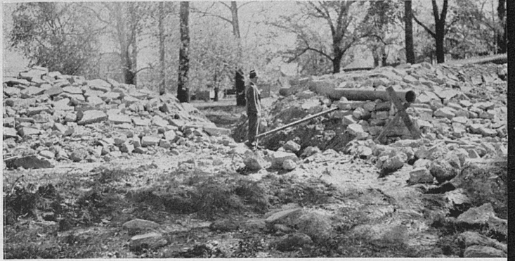
Both these dams failed because of faulty construction. That at the left settled too much at one point and then washed out; that at the right was destroyed by overflow when the spillway, built too small, failed to carry off the surplus water.
