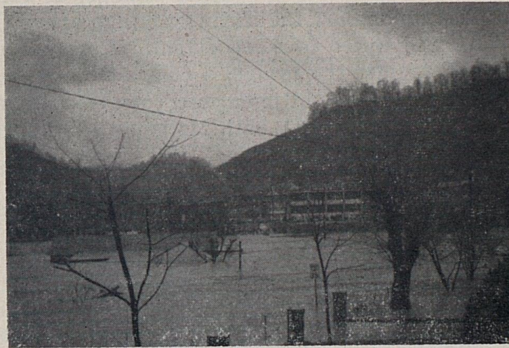
FLOOD WATER AT HYDEN
