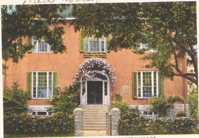
GUEST HOUSE OF HISTORIC SHAKER VILLAGE.
