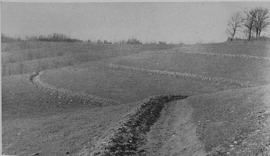
Diversion ditches on sloping pastureland help to control erosion if sod cover becomes thin.
