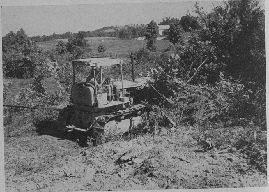
Bushes and trees may be cleared off the land with a bulldozer.
