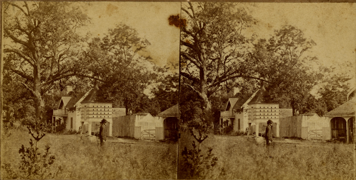
10. Ashland - Cottage & Pigeonhouse
