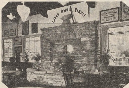
The Fountain in Dicker Hall
